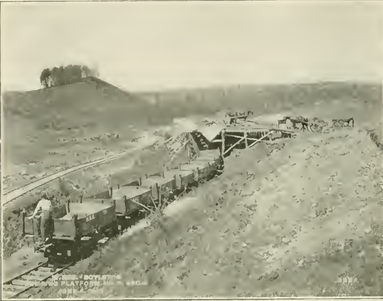
LOADING AND DUMPING PLATFORM.
